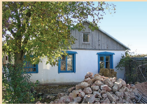
The Ryabushev home, built by HH building teams
